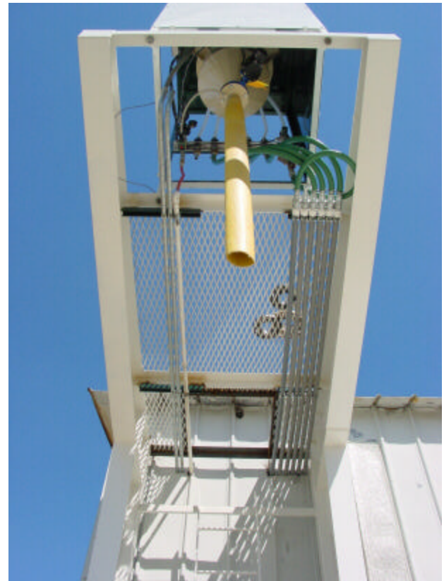
DISCHARGE INTO TRUCK
